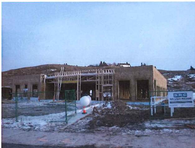
Parapet Framing
