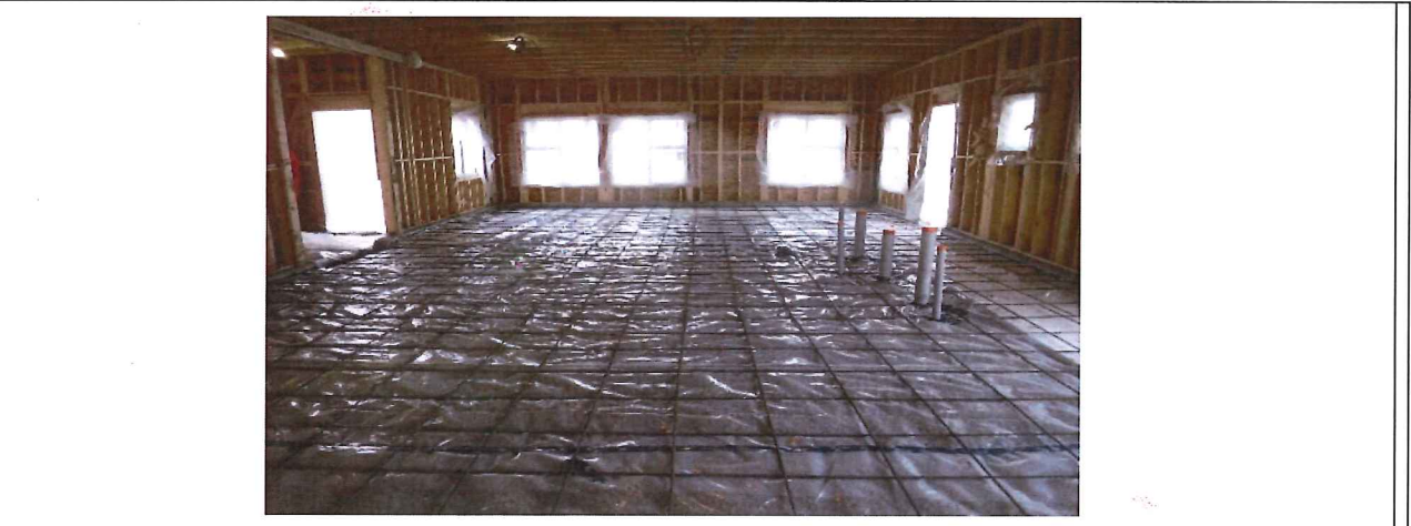
Rebar for Slab and Radon Membrane
