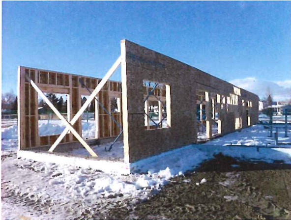
Wood Frame Wall Installation
