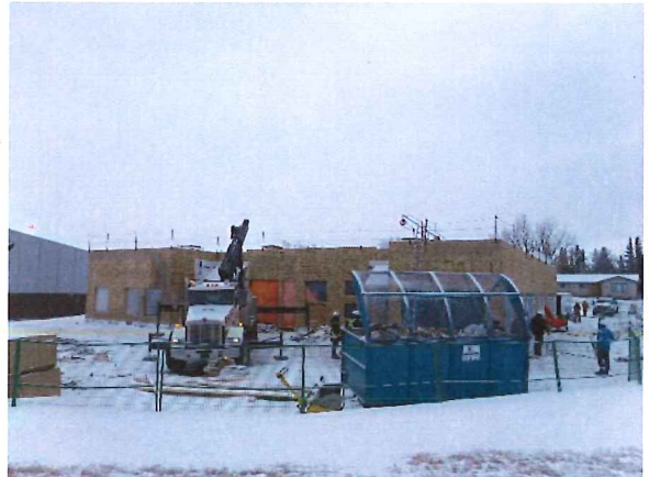
Roofing Material Delivery
