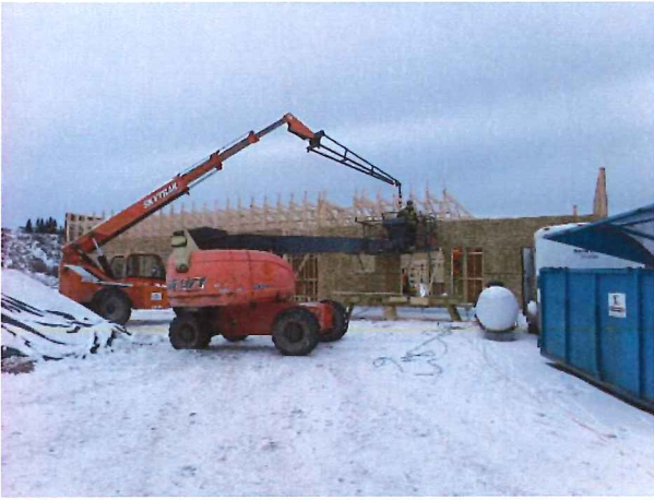
Roof Truss Installation
