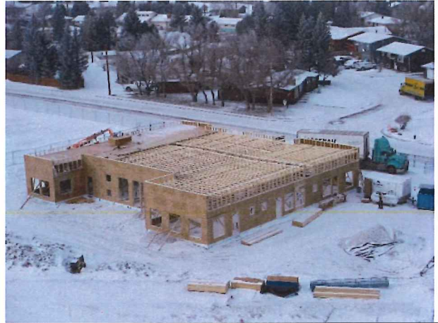
Roof Sheeting Underway
