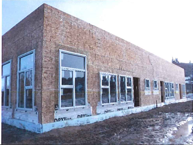
Window Installation (Exterior)
