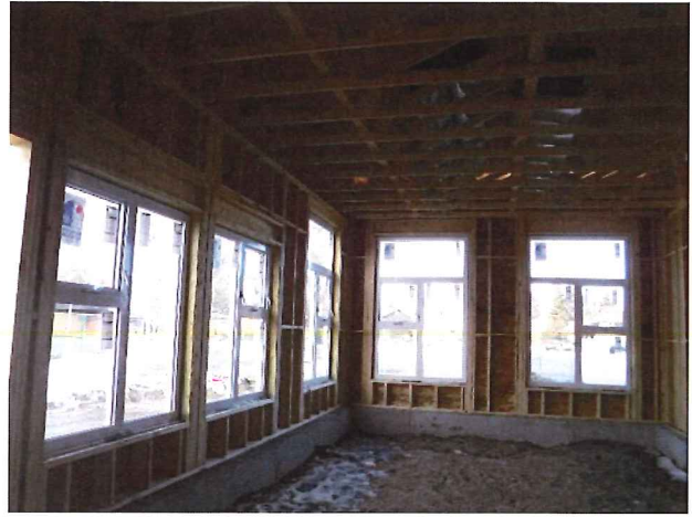
Window Installation (Interior)
