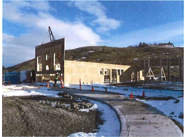
Wood Frame Wall Installation
